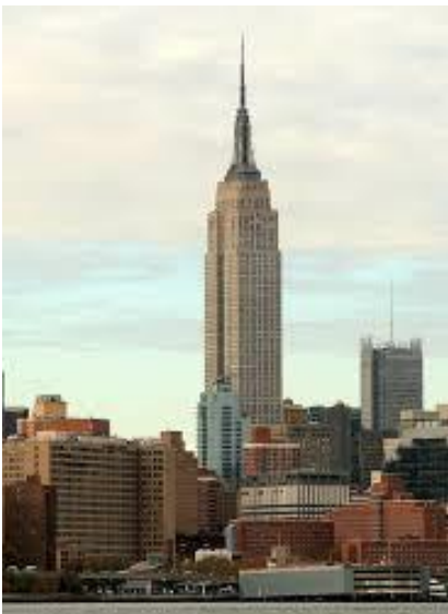
The Empire State Building, 1931 (Art Deco) (ArchDaily.com)
